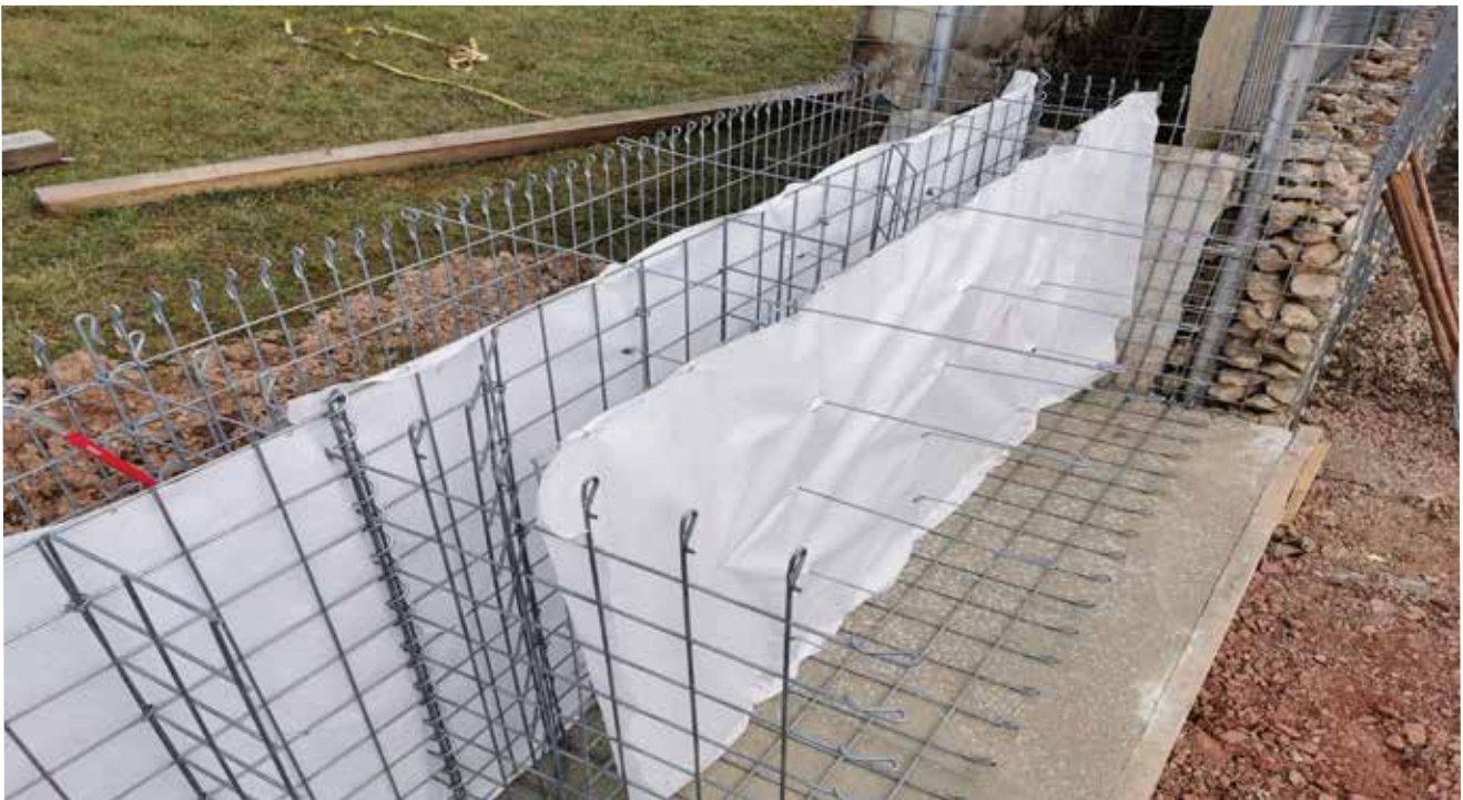
Image: Assembly of the first layer, connecting the formwork grid
