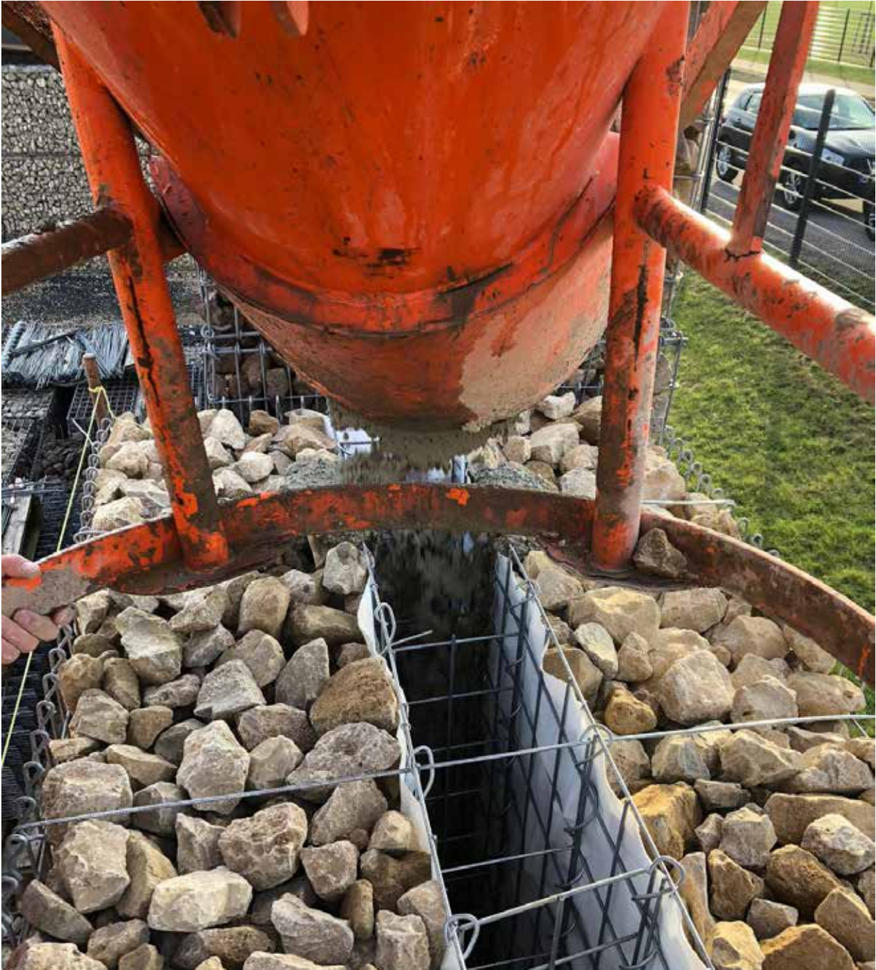
Image: Filling with concrete
