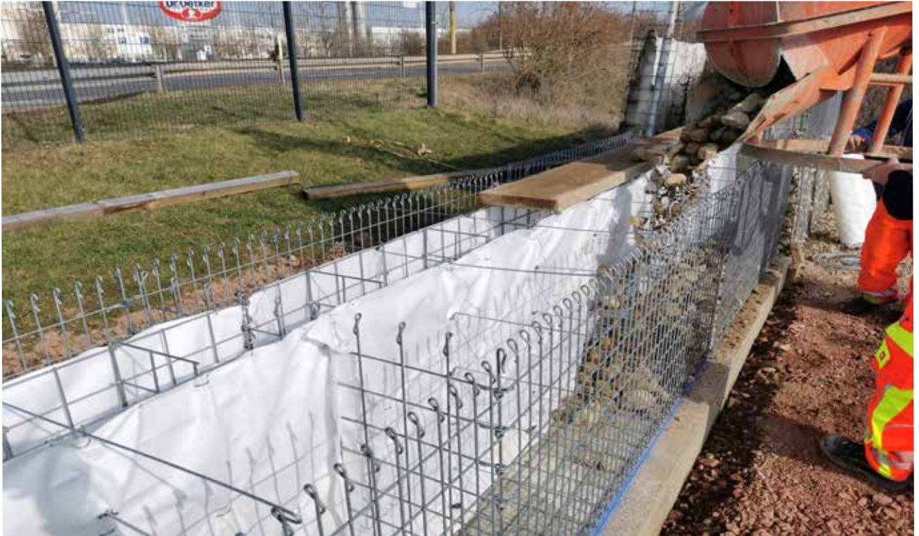
Image: Filling the first layer with stones
