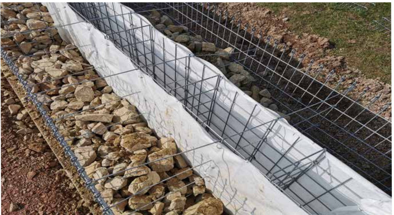
Image: Partial filled Silent R® - noise protection gabion
