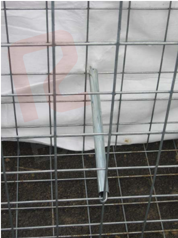
Diagram: Correctly assembled spacer with spacer tube
