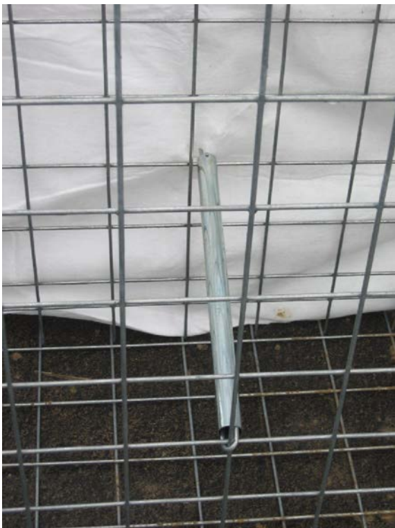
Diagram: Correctly assembled spacer with spacer tube
