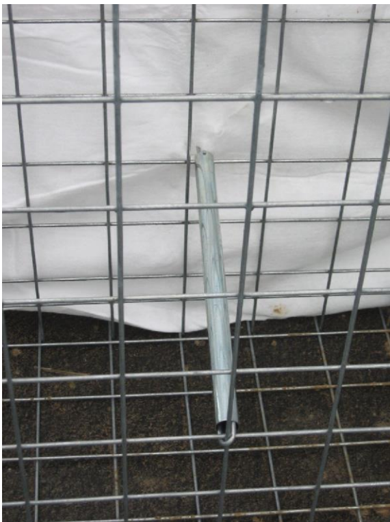
Diagram: Correctly assembled spacer with spacer tube
